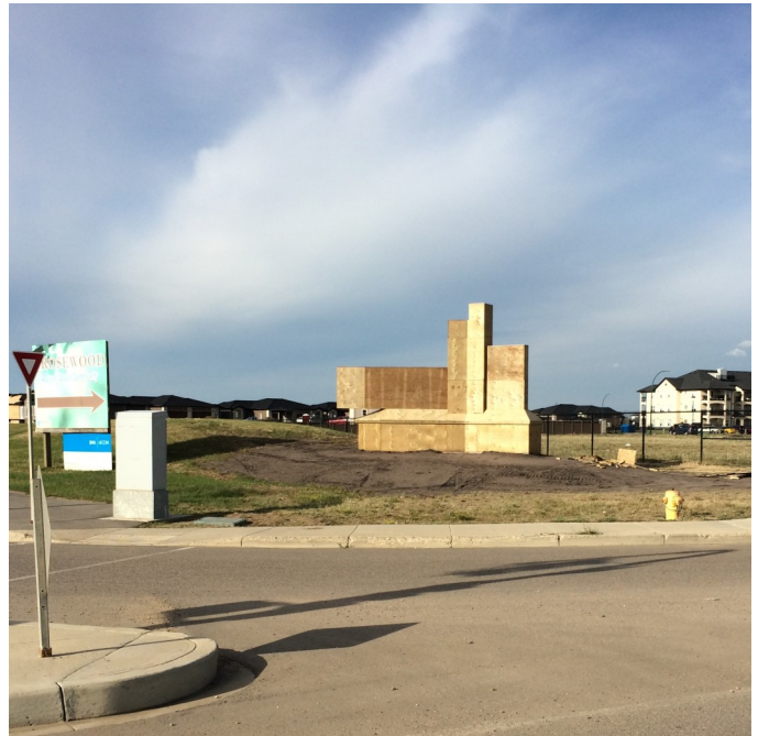
Rosewood entrance sign construction August 2015
