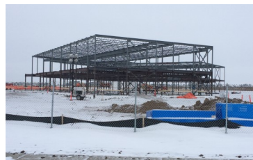
Rosewood Elementary Schools Construction Site February 2016
