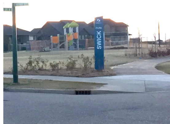
Swick Park Construction nearing completion
