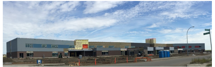
Rosewood Elementary Schools Construction Site May 2016
