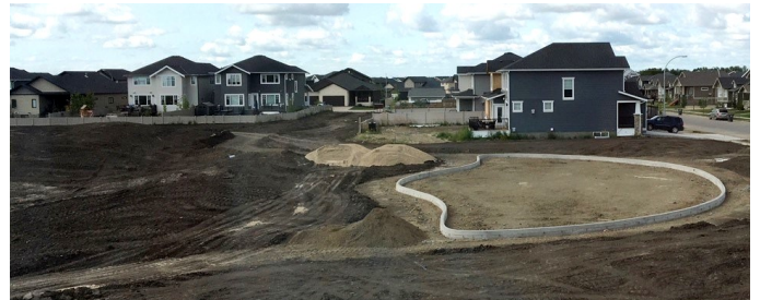
Struthers Park Construction - Summer 2018
