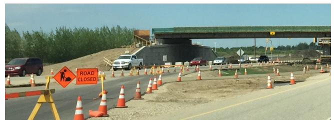
Boychuk Drive / Highway 16 Interchange Project Construction Tentative Completion July 31, 2019
