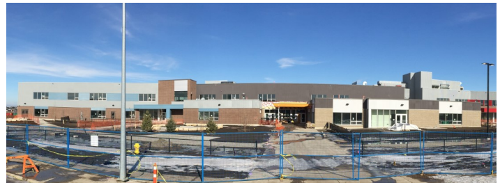
Rosewood Elementary Schools Construction
