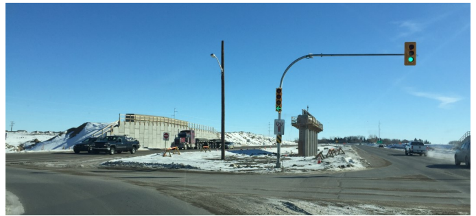
Boychuk Drive / Highway 16 Interchange Project Tentative Completion July 31, 2019
