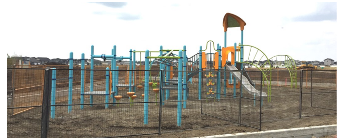
Glen H. Penner Park Construction - Fall 2017
