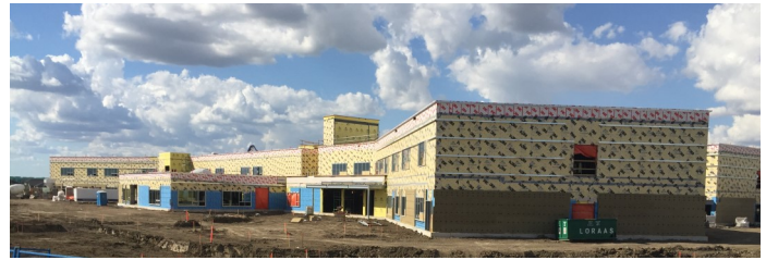
Rosewood Elementary Schools Construction Site May 2016
