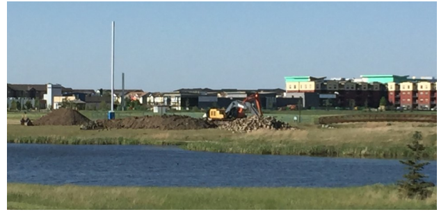
Hyde Park Naturalized Area Weir Construction - May 2016
