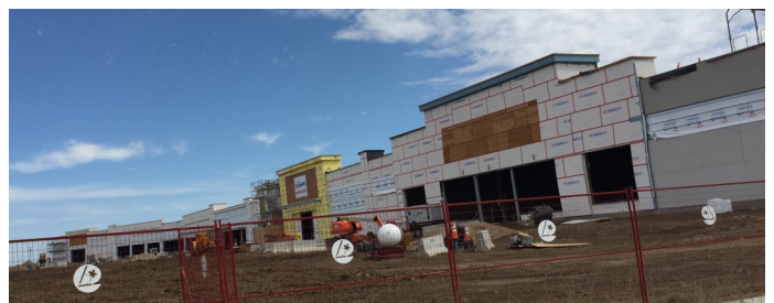
Rosewood's Meadows Market Construction - Spring 2018
