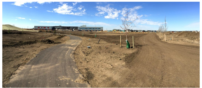
Glen H. Penner Park Construction - Spring 2018
