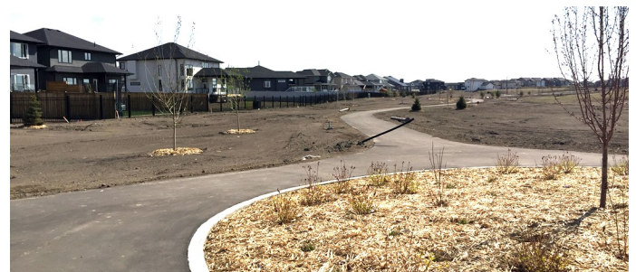
Mackay Park Construction - Spring 2018
