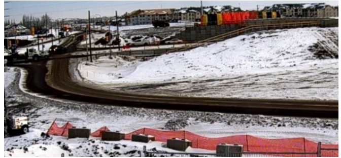
Boychuk Drive / Highway 16 Interchange Project Tentative Completion July 31, 2019
