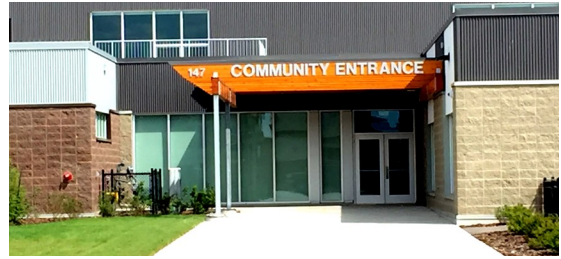
Rosewood Community Centre Community Entrance 147 Olson Lane West
