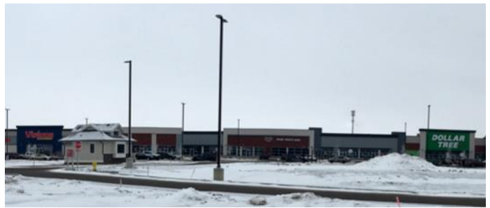
Rosewood's Meadows Market Construction - November 2018
